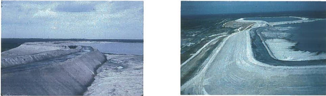
Fig 3. (a) Elevated sloping rim ditch; (b) Beaches formed from rim ditch cuts
