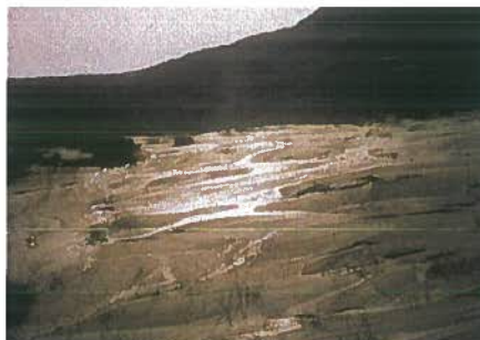
Fig 10. Seepage from base of dry stack
