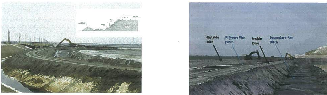
Fig 4. (a) Upstream method of construction; (b) Equipment accessible inner & outer dikes;
